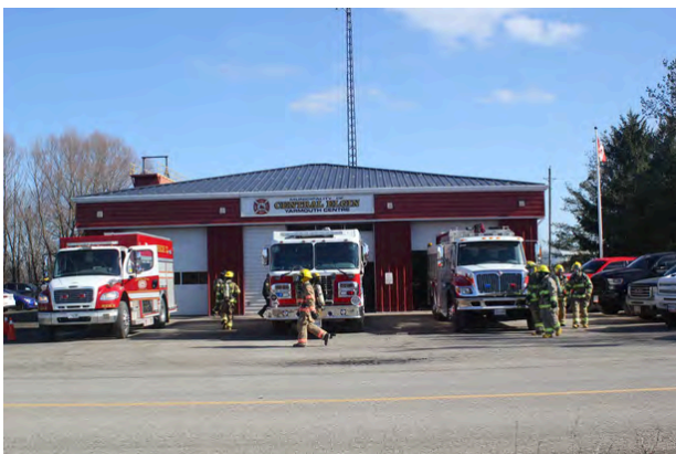
Fire Station 3 - Yarmouth 9538 Yarmouth Centre Road
