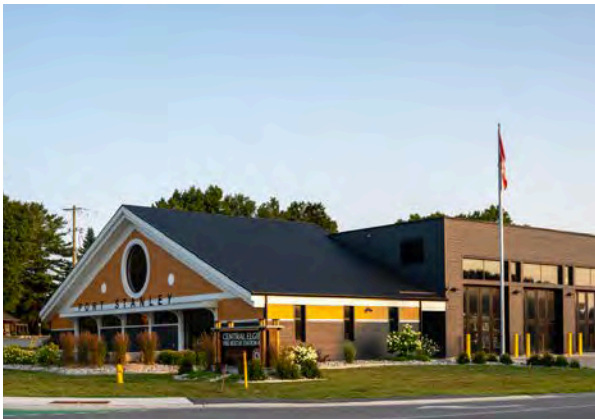
Fire Station 1 - Port Stanley 218 Joseph Street
