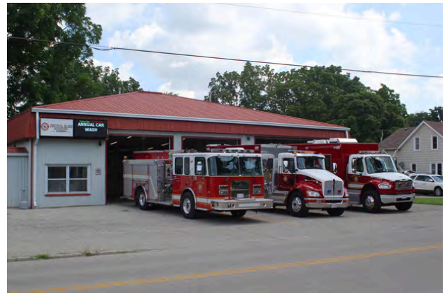
Fire Station 2 - Union 42702 Sparta Line, Union
